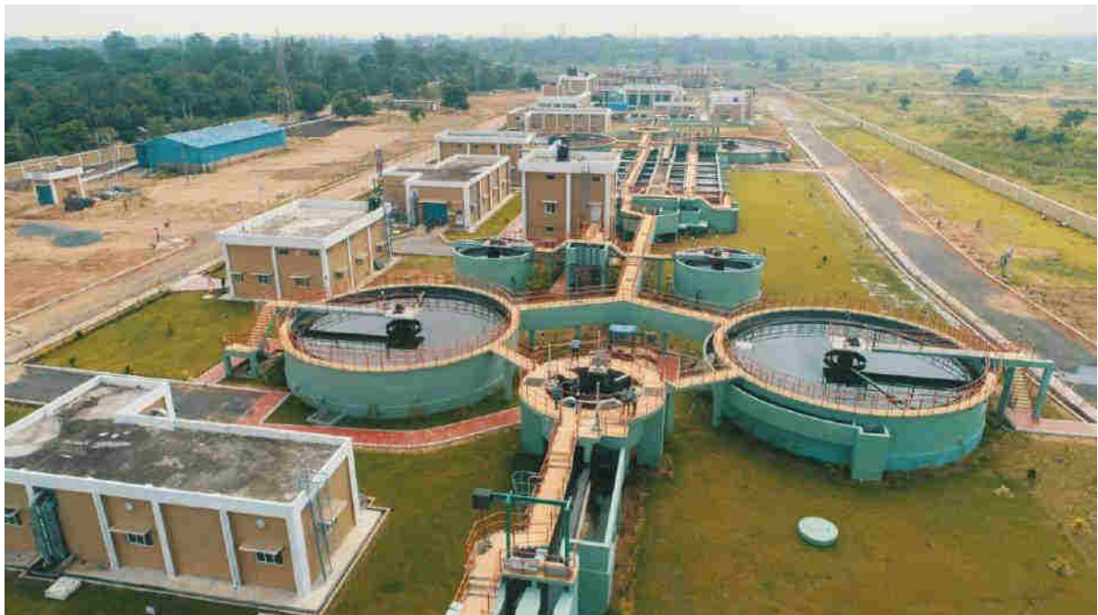
16 MLD STP at Mattagajpur Cuttack
