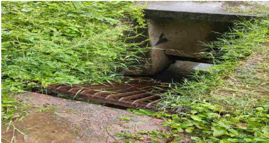
33 MLD STP at Mattagajpur Cuttack
